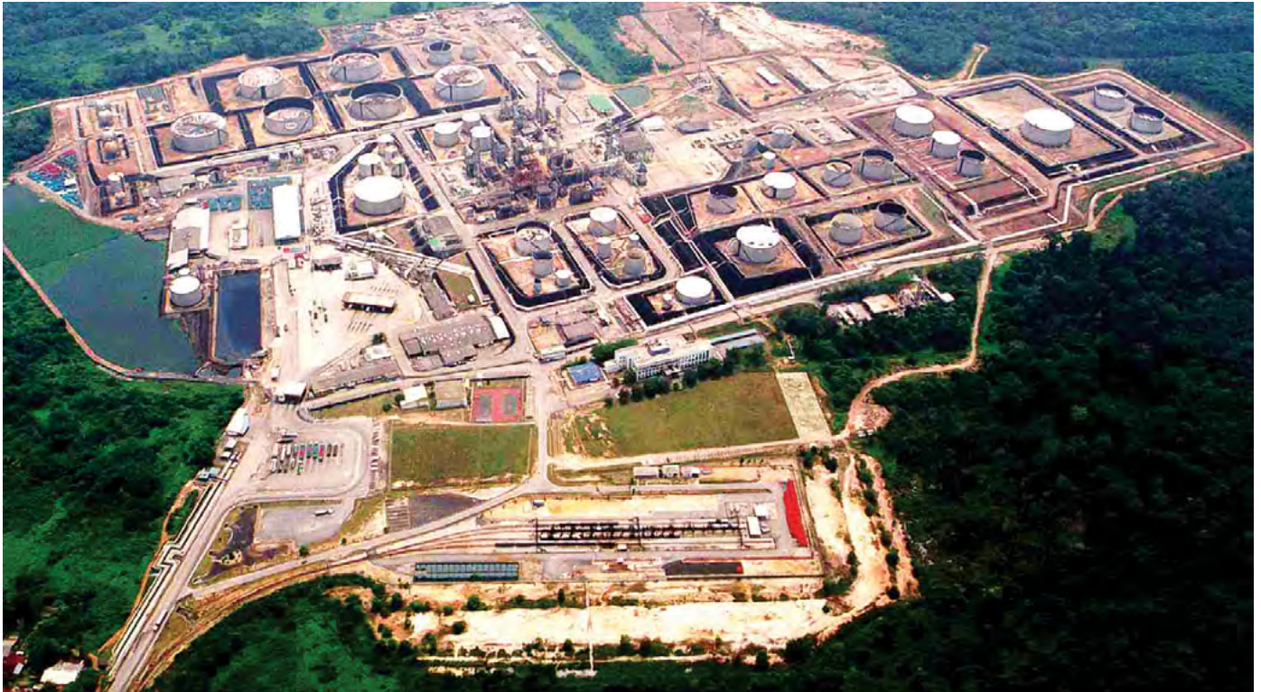
> Aerial view of Port Dickson Refinery
