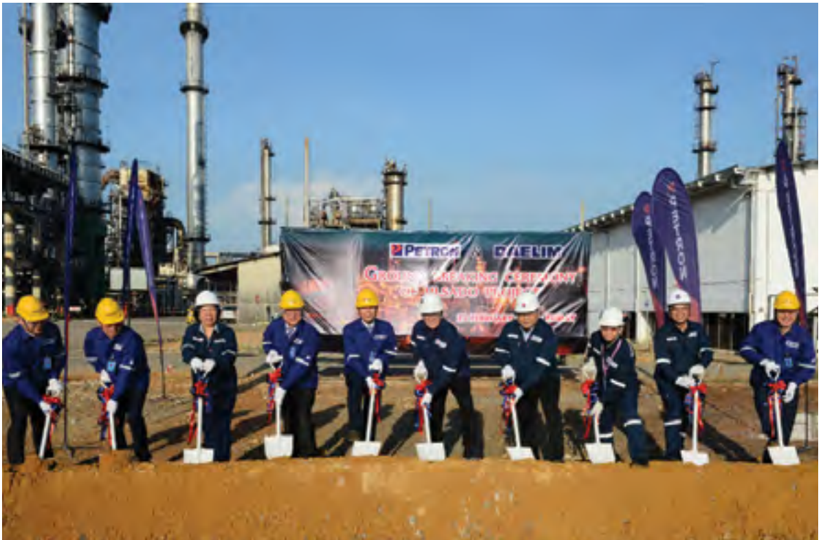
Groundbreaking of Diesel Hydrotreater mark the beginning of the project
