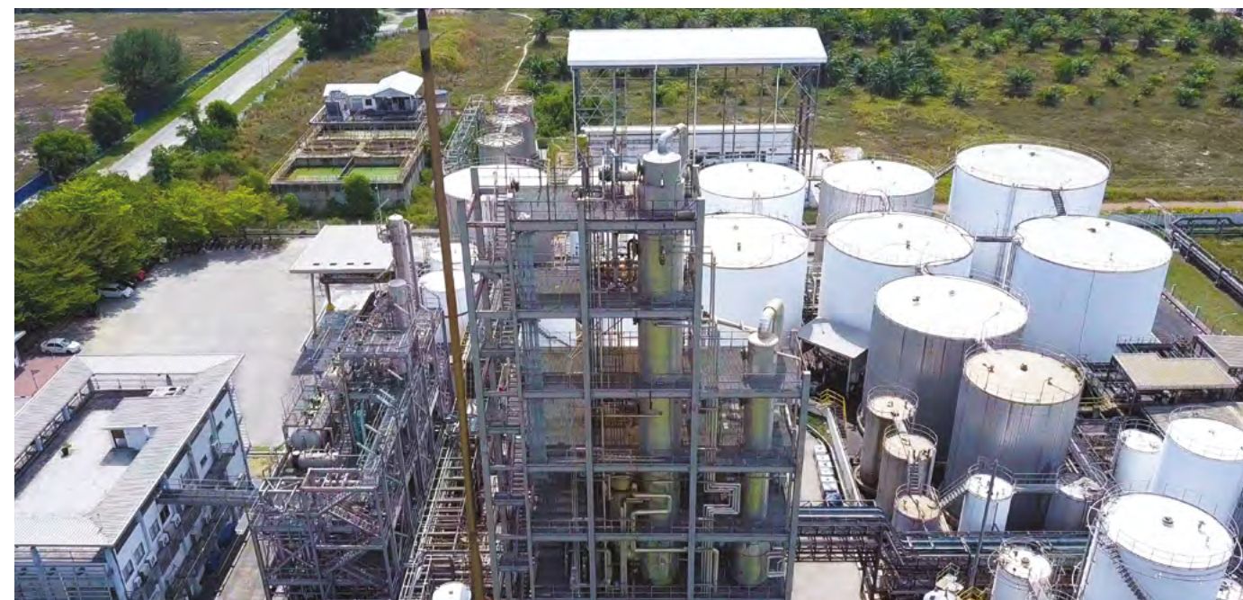
Lumut PME Plant supports the production of biodiesel fuel.
