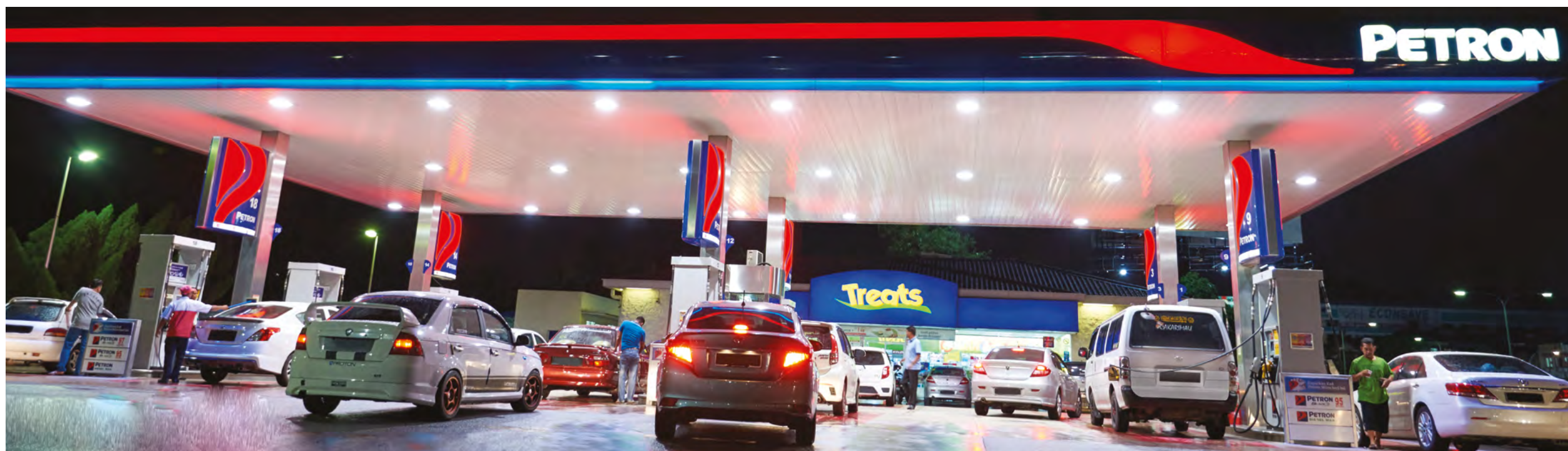
Our stations and Treats stores throughout the country are always ready to serve the needs of travellers.
