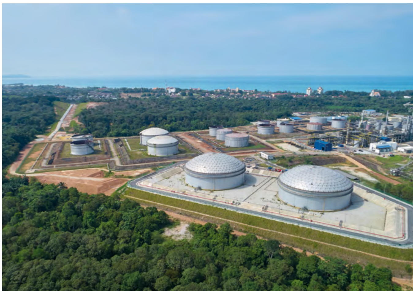
● The Marine Import Facility 2 connects the offshore facility through 1.5km of pipelines to two-250 kb tanks.
